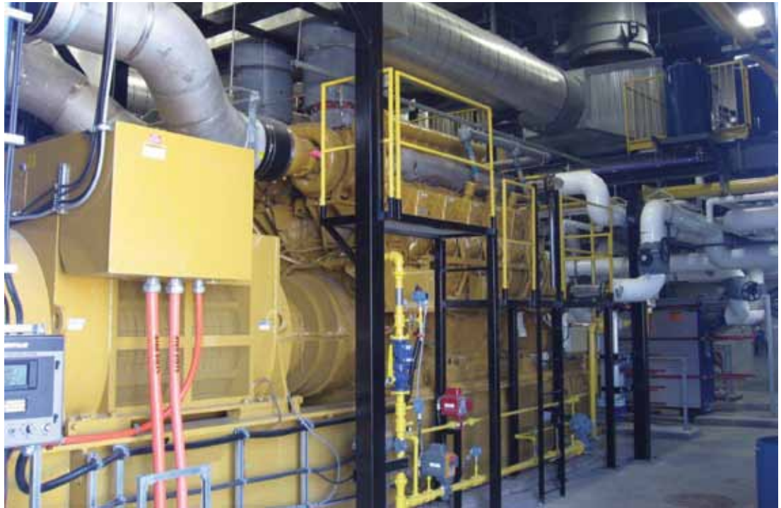
Photo : Markham District Energy Inc.
